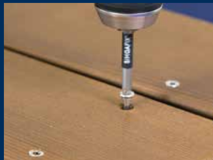
3. Screw in the new screw
