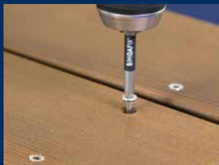
3. Screw in the new screw
